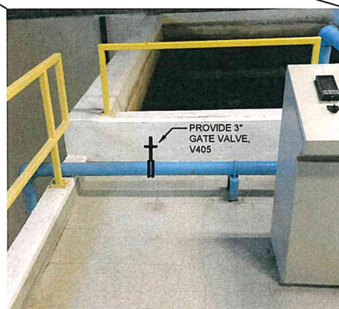
GATE VALVE, V405 DETAIL 1 NTS
