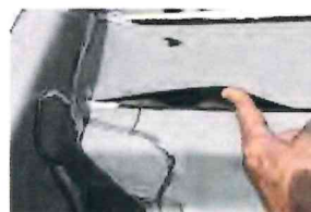
Edge Detail Inspections / Repair
