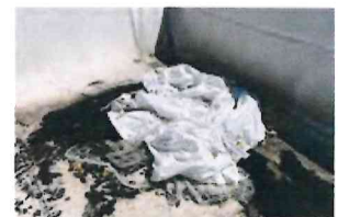
Debris Removal and Cleaning
